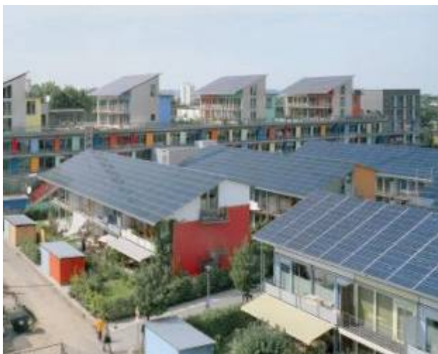
View from south-east showing the PV-roofs (copyright ©2007: Solarsiedlungs GmbH)
