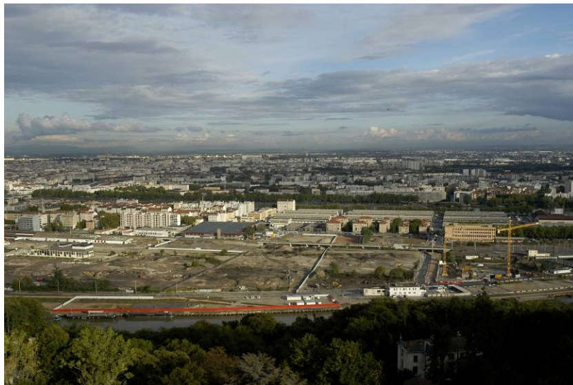
Lyon-Confluence area First housing buildings under construction
