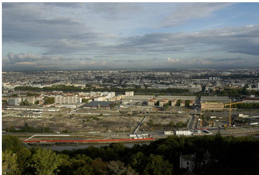
Lyon-Confluence area First housing buildings under construction
