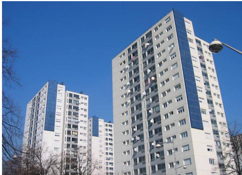
La Darnaise district PV modules were optimised in order to limit mutual shading
