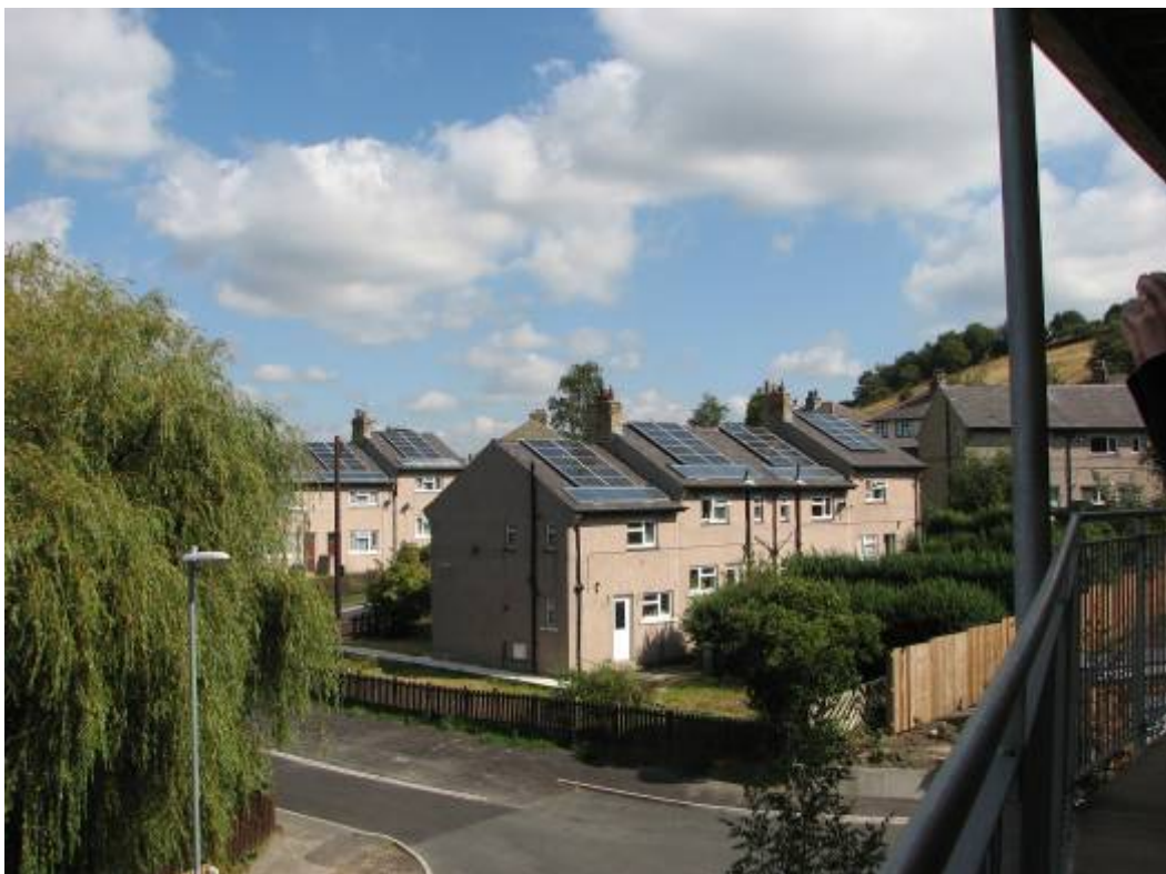
PV and Solar Thermal retrofit to houses in Primrose Hill
