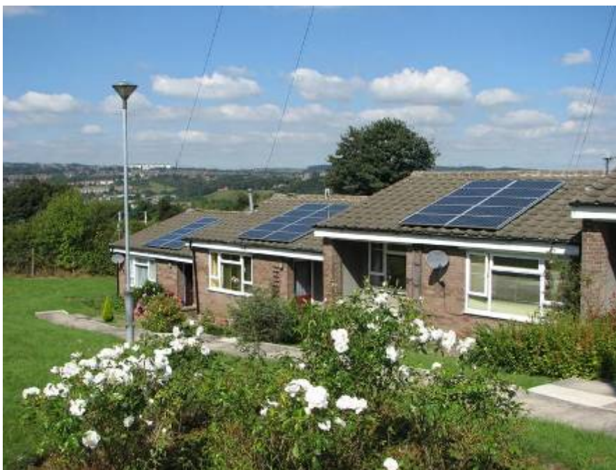
Fernside solar village housing
