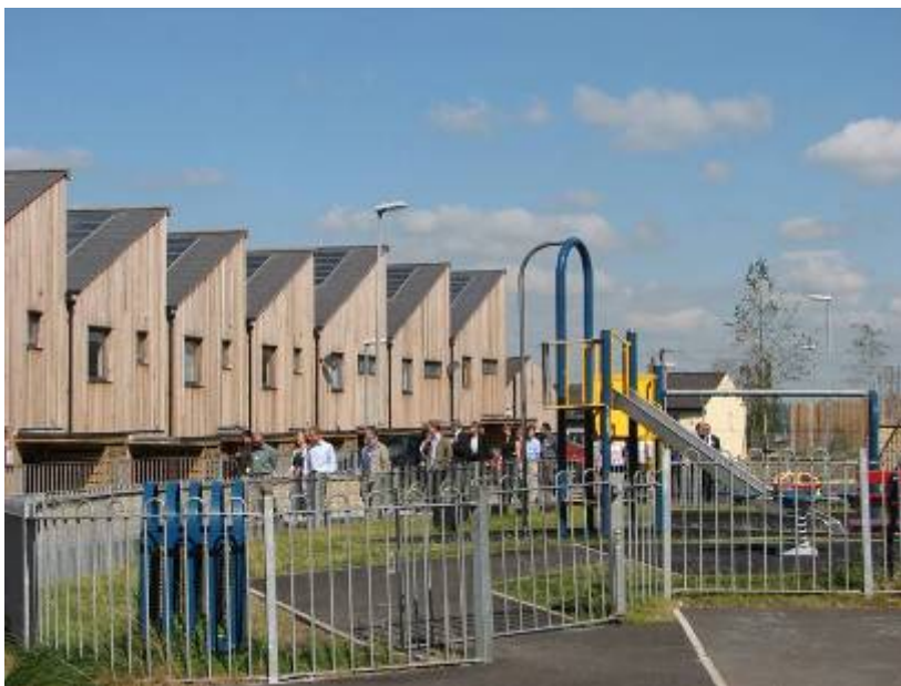
PV on new housing at Primrose Hill
