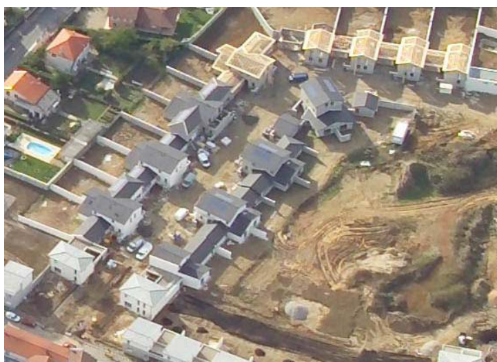
France-Terre detached houses PV systems with different orientations
