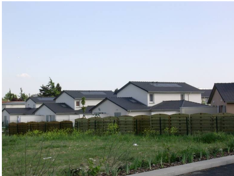
France-Terre detached houses 1 kWp integrated PV system each
