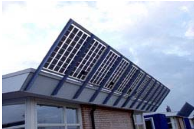
Subproject: Dyke or noise wall houses, © Photographer: Astrid Schneider, Berlin
