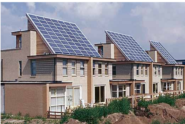
Subproject: prefab PV roofs, Photo: © NOVEM
