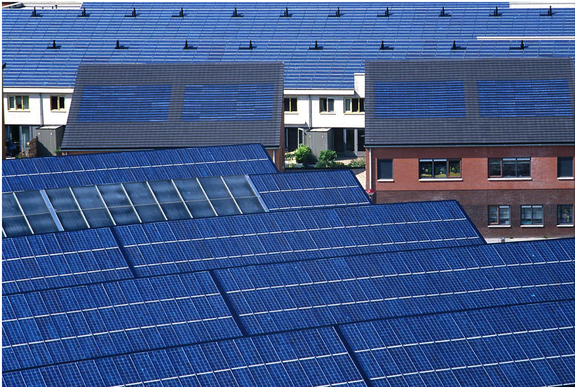
Figure 1: View from the south of the sports hall roof, also showing the school houses and the first row of housing (Photograph R. Schropp)
