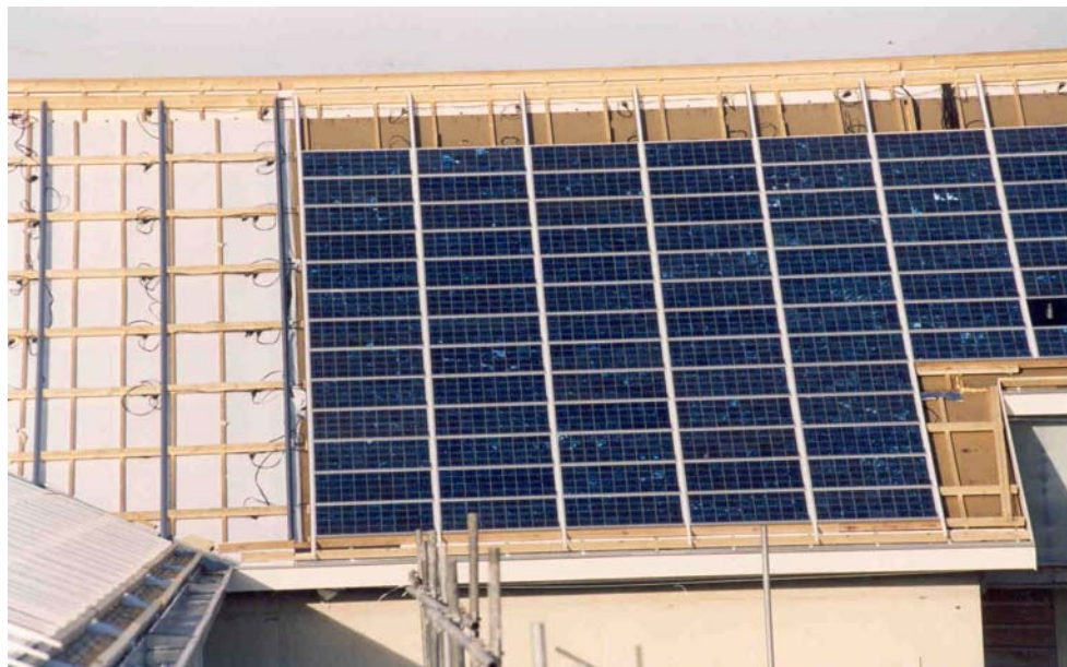
Photo 3: Mounting of the PV modules
