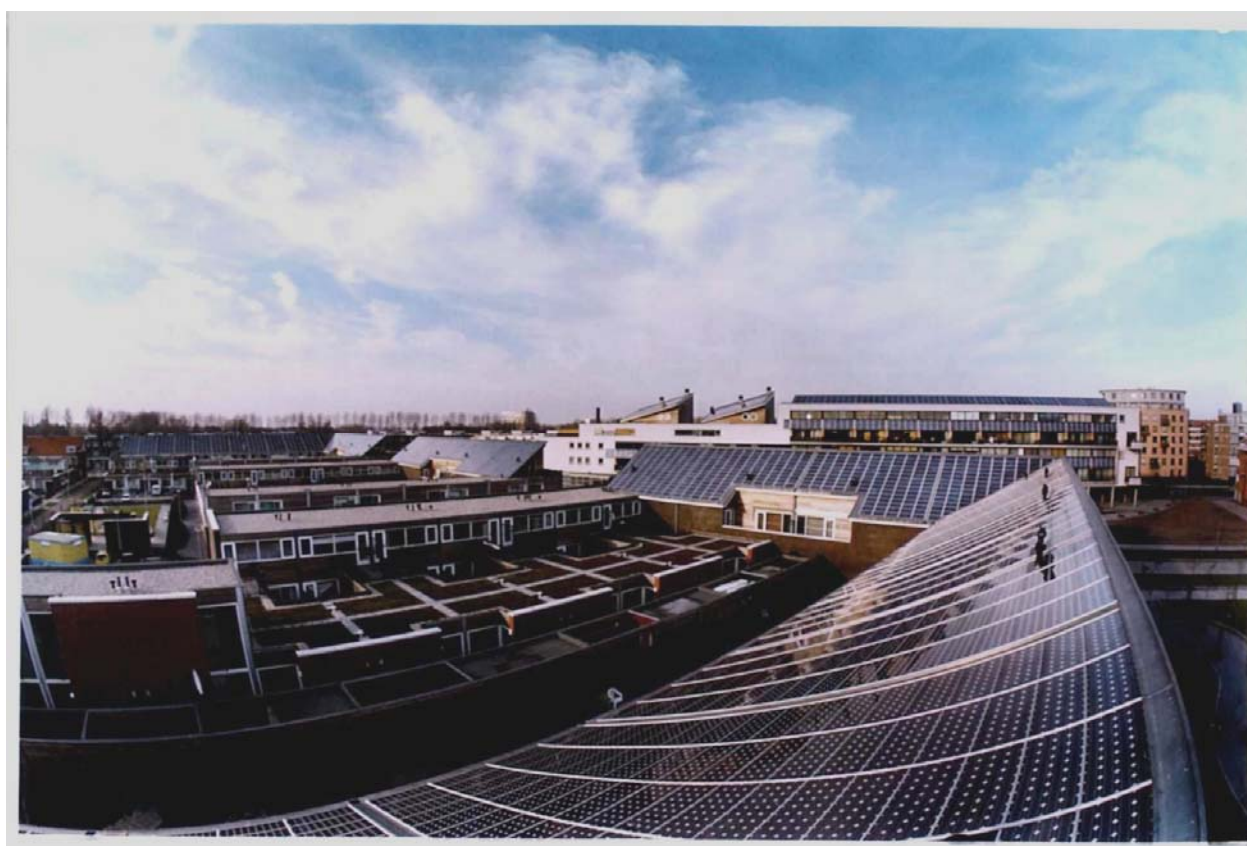
Photo 2: Wide angle photo of the Nieuw Sloten PV houses. In the foreground is the west facing roof, in the centre is the south facing roofs and in the background the apartment building with PV facade and two penthouses with angled roofs. To the left the east roof can hardly be distinguished.
