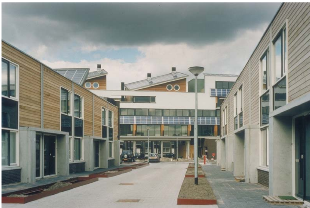
Photo 1 - View from the South of the apartment building with 2 penthouses with PV roofs
