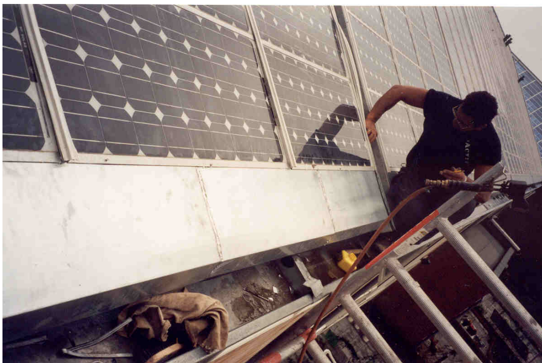
Photo 6: The edges of the roofs were finished with aluminium plates.
