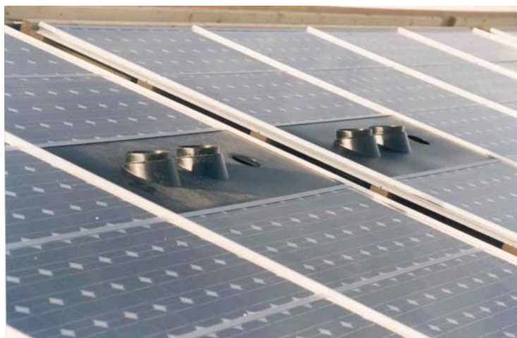
Photo 5: Plates for the integration of chimneys and ventilation pipes
