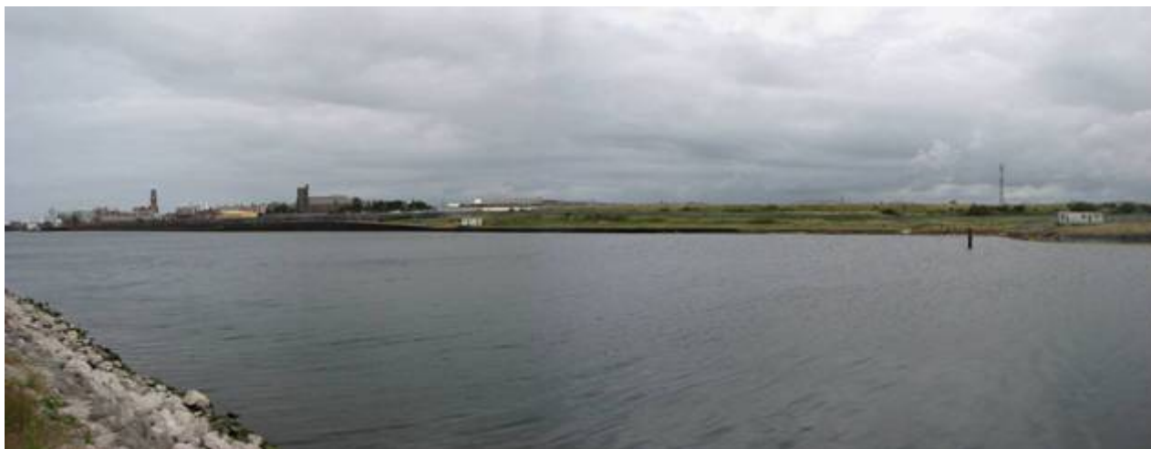
Photo 4: View of the Marina Village Housing site from across Ramsden dock, a new waterfront will be created with shops, restaurants and housing
